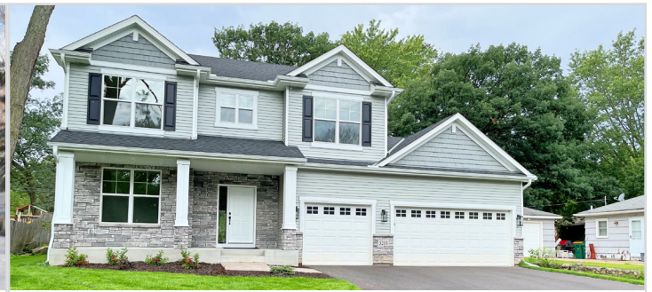
5213 Pennsylvania Ave N - After
